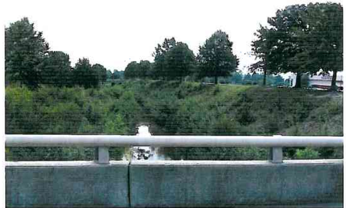
Rocky Creek Before
