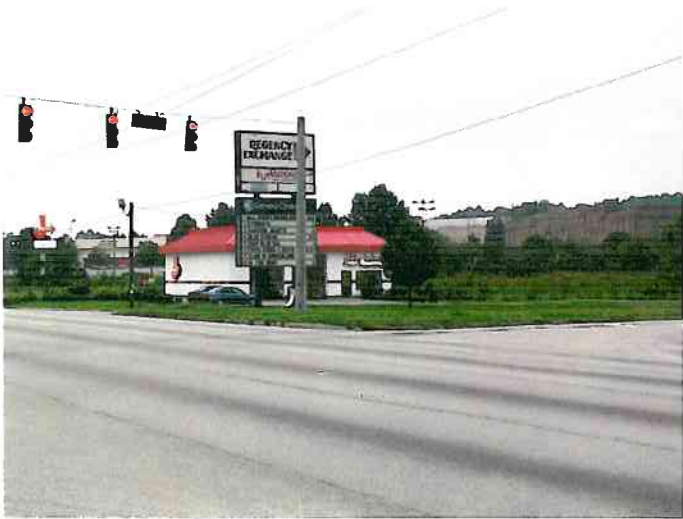
Rocky Creek Before
